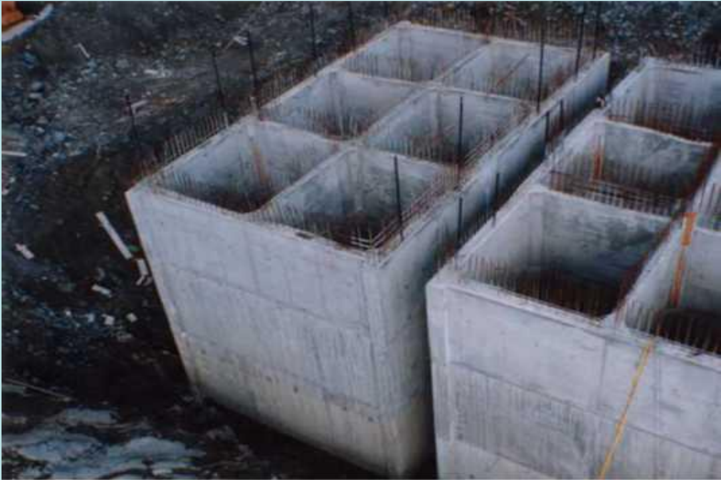
1000te Reinforced Concrete Caissons for RoRo Terminal- Rosslare, Ireland
