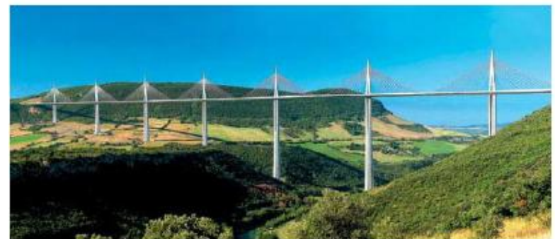
Substructure here is expensive compared with superstructure
