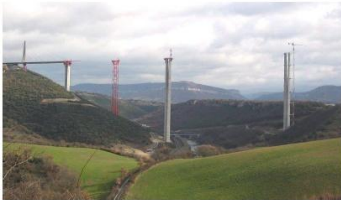
In the Millau Aqueduct, the superstructure was completed inland and pushed into the span
