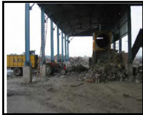
Lahore compost plant
