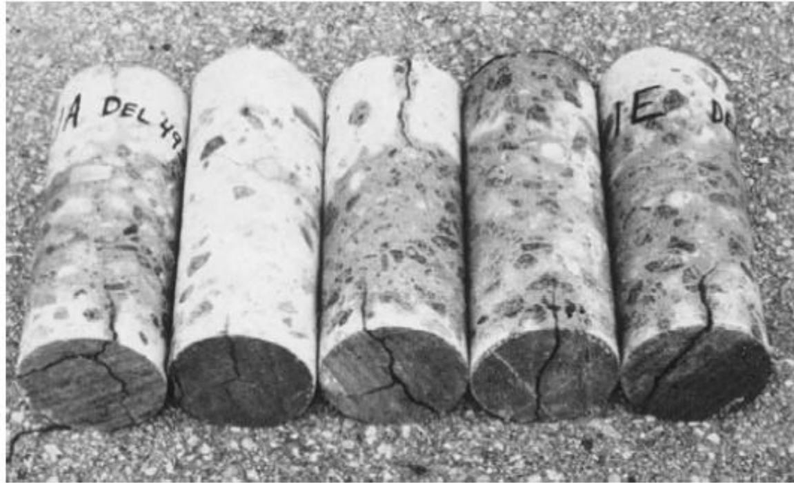
Pavement Cores Vertical Cracking
