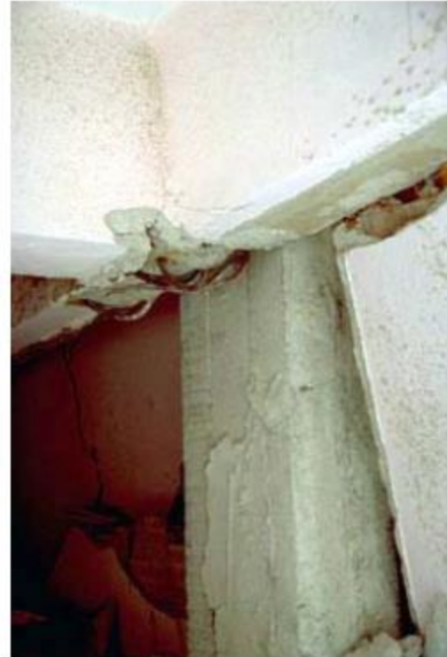
Figure 3-32 Damage and failures at ends of moment-frame columns
