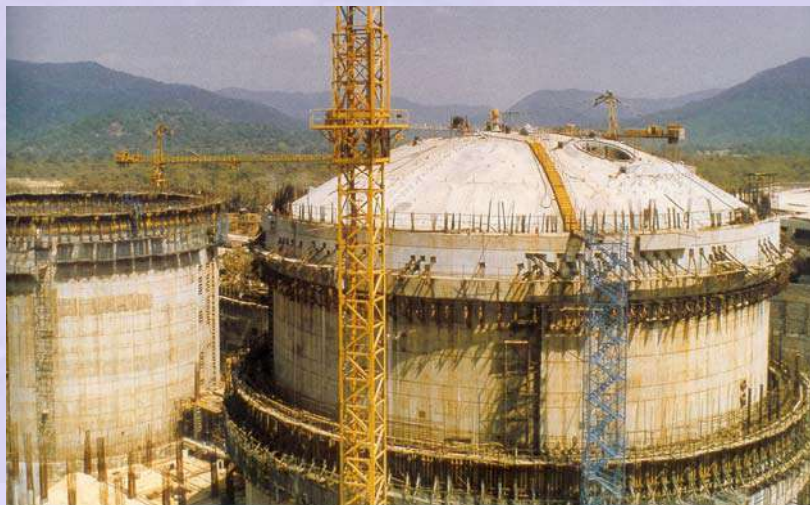
Figure 1-2.7 Circularly prestressed containment structure, Kaiga Atomic Power Station, Karnataka
