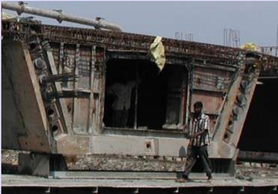
Figure 1-2.5 Post-tensioning of a box girder (Courtesy: Cochin Port Trust, Kerala)
